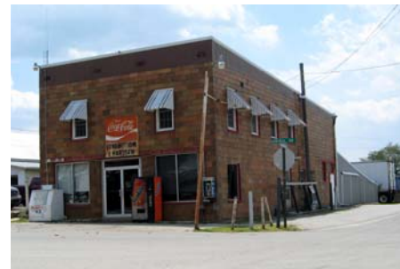
Commercial building in Central
